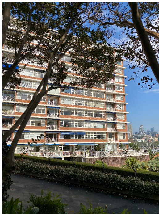
Figure 2 Glenhurst Gardens, Darling Point, by Douglas Forsyth Evans. Completed in 1959, it is a notable early large-scale linear apartment building in Sydney. (Source: GML 2024)
